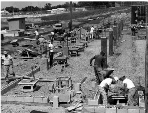
Workers lay the foundation for John D. Sulsberger Memorial Stadium on July 19, 1964. (Photo: Times Recorder file photo)
